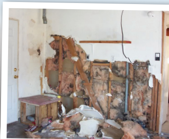
mold, damaged drywall/insulation
