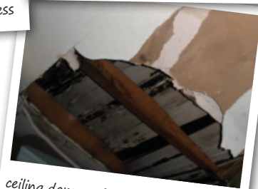
ceiling damage from water leak above
