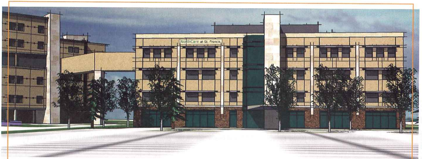
The London Real Estate Group is currently building Northcare, a $15 million, 80,000-square-foot medical office building in Colorado Springs, Colo.
