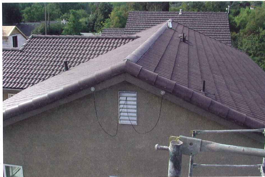
Twelve color-matched cool and hot coatings (top) of the type used on a demonstration home in Sacramento, Calif. (bottom)
